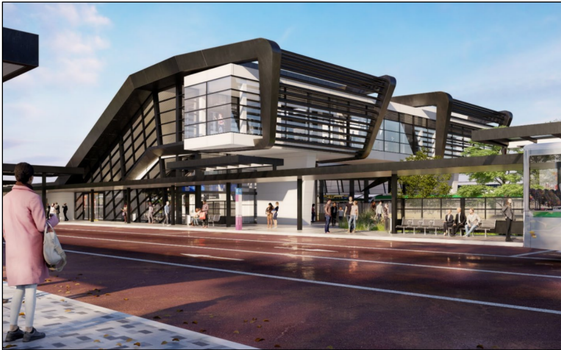
Figure 18: Nicholson Road Station 61
