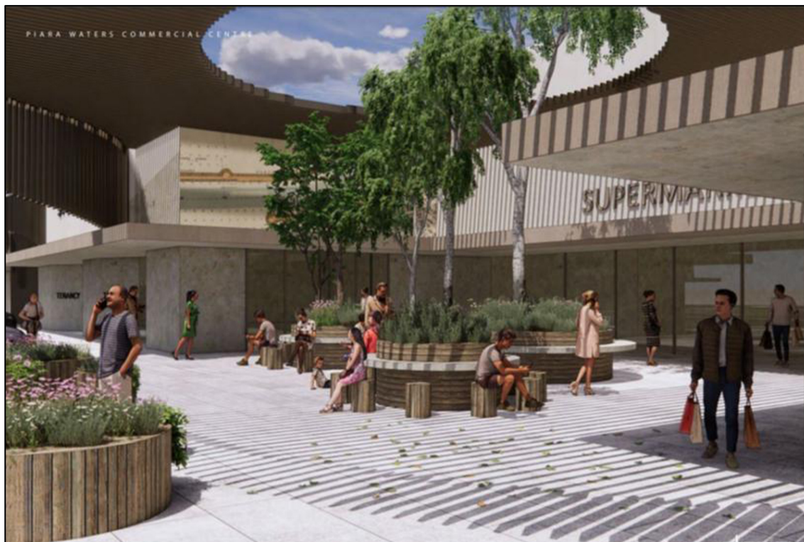
Figure 19: Piara Waters Shopping Centre
